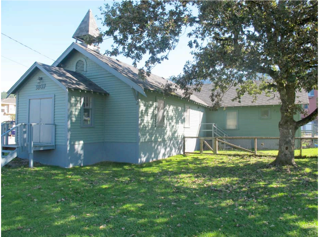
The original United Church building and its rear addition
