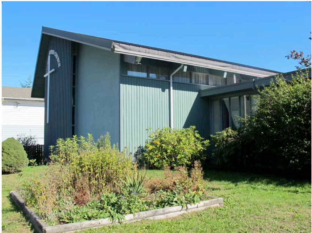
The 1963 Christian Education Centre Building
